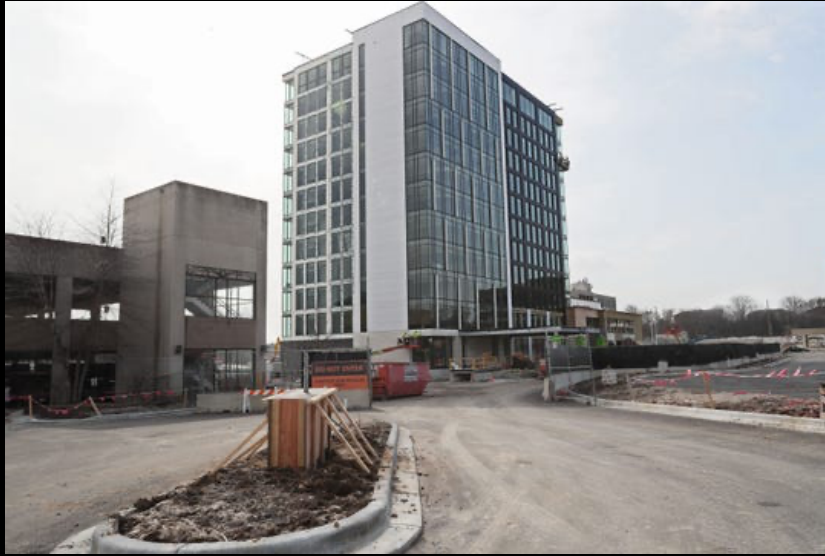
New Renaissance in Wauwatosa (Milwaukee) opening in August
