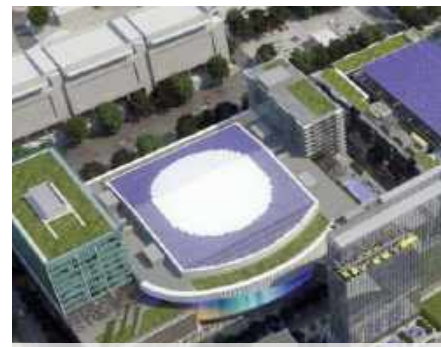
Richmond, VA Downtown Arena Mix
